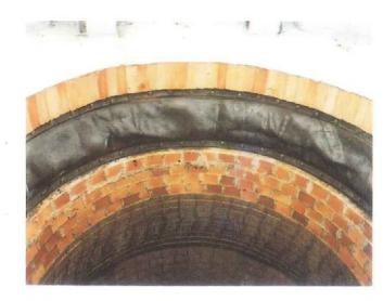
Connection with the acid-resistant inner liner and cross joints can be executed in various ways.
