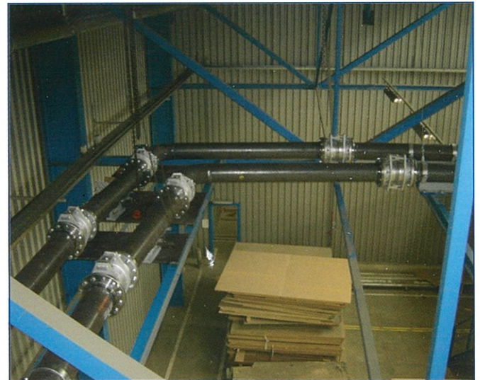
3 pin 'hinged' expansion joint system to absorb large movements of the piping, without transmitting pressure thrust loads on adjacent pipework. This solution is ideal for suspended piping, where it can be difficult to position sufficiently strong fixed points.
