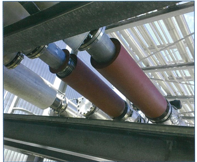
Axial expansion joint (DN200) for large movement absorption, comprising several bellow elements and equipped with movement limit rods and outer shroud for protection against mechanical damage and directional guidance.
